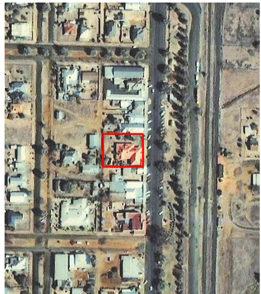
Site No. 18 Multi Purpose Building - Dunedoo
